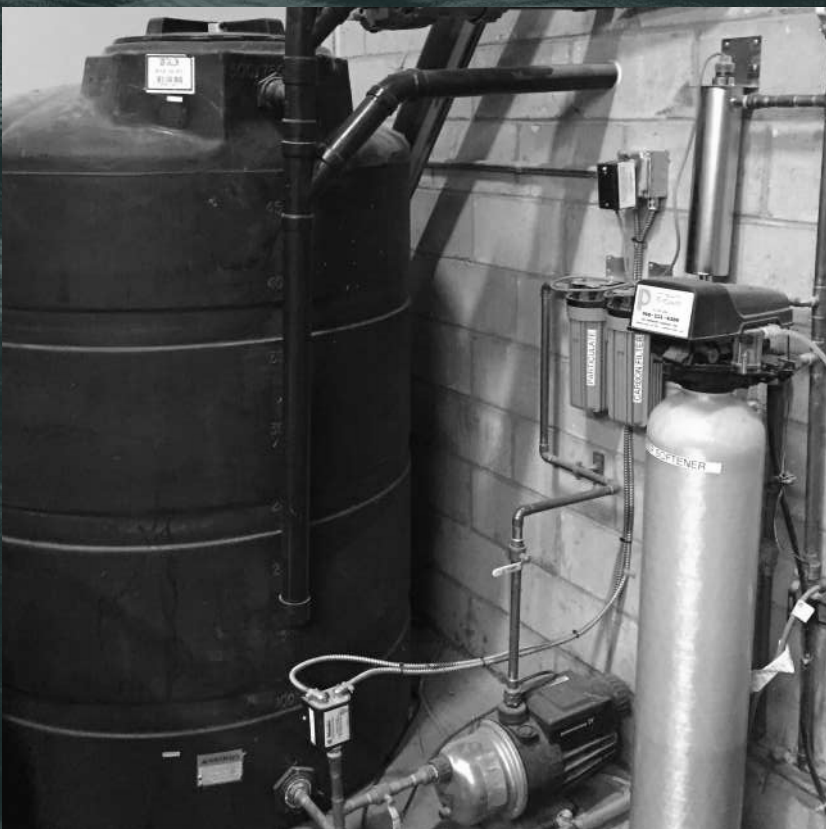
This rainwater capture system we installed at our Piscataway facility captures 100% of the water required for production.
